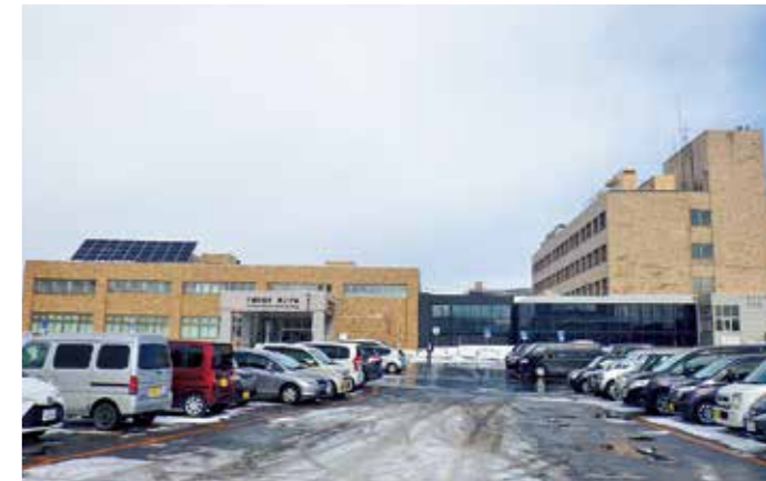
千歳市役所本庁舎(右)と第2庁舎(左) Chitose City Hall Main Government Office (right) and Second Government Office (left) / 千岁市政厅主厅舍(右)及第2厅舍(左) 치토세시청 본청사(오른쪽)와 제2청사(왼쪽) / สำนักงานเทศบาล
